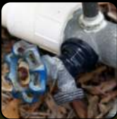
Repairs loose or leaky plumbing
