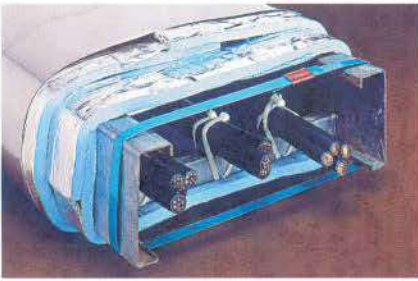
To meet Ashland's needs, 0.3" thick blankets were provided, cutting installation time
