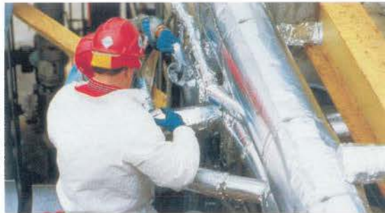
Installing the ceramic mat insulation on the complex conduit lines at Ashland's St. Paul plant was hastened by the ability to cut and fit the material with common tools
