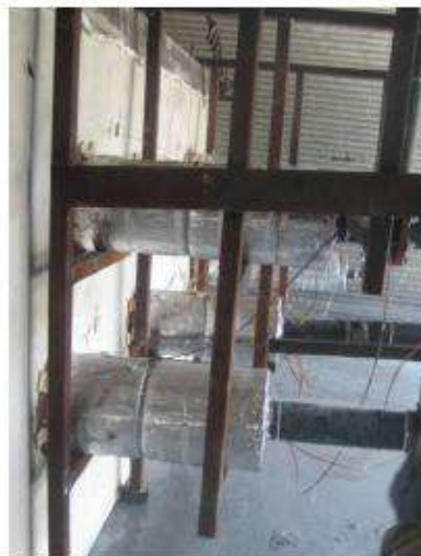
Figure 4-7 Side View of Unexposed Side Following Hose Stream Test
